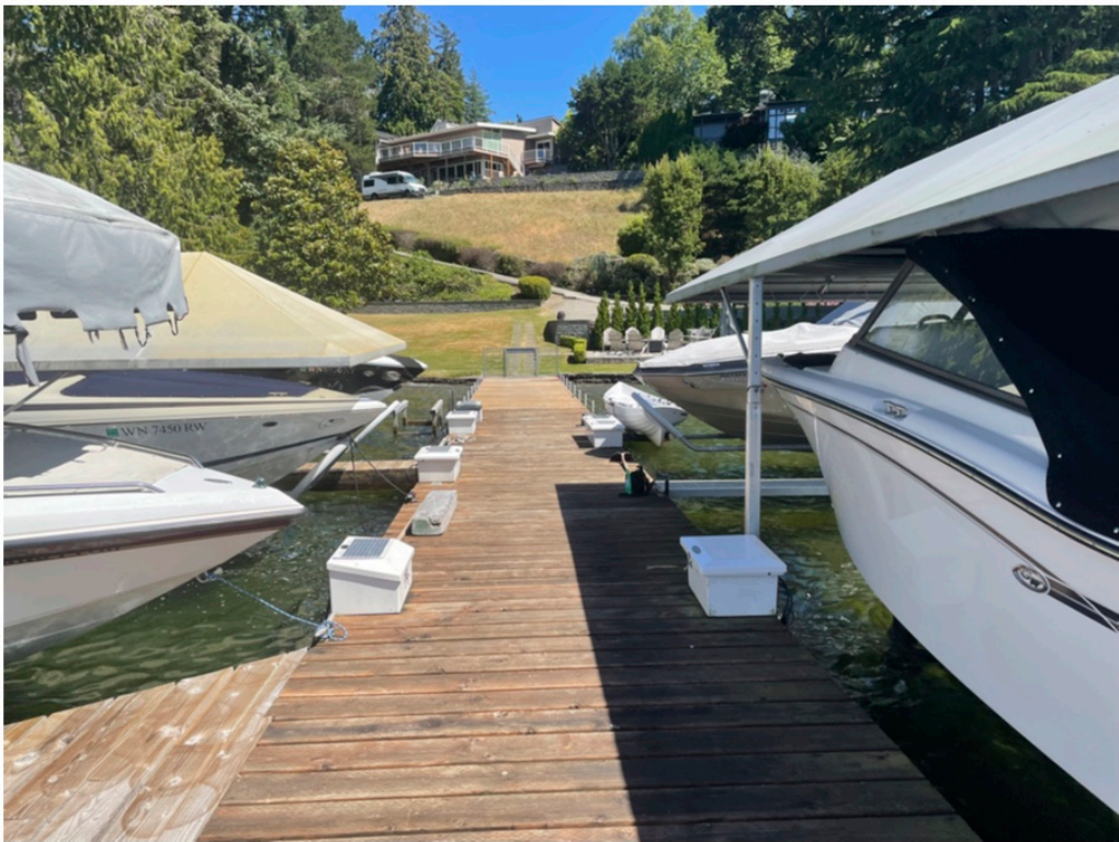
Photo 2 -Existing dock looking landward.
